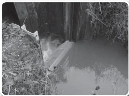
*One of the weirs in the river floodbank permitting water to flow onto the grazing marsh.*
